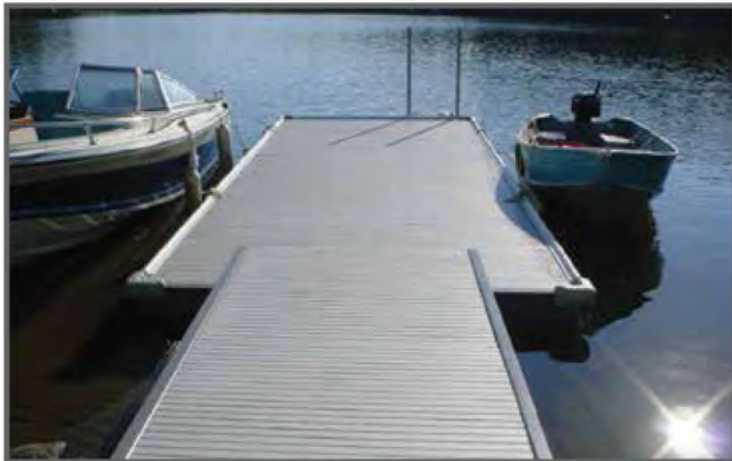
This all FRP dock was designed for a private lake front residence in Canada and utilized barefoot friendly, ADA compliant Aqua Grate® pultruded grating and Dynaform® support beams.
