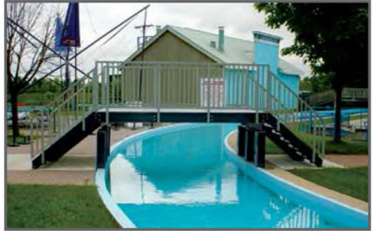
This bridge at a waterpark was constructed using ZeAllgrate's railings, grating, stair treads and structural shapes. In addition to being ADA compliant and slip resistant, this grit-top surface is also barefoot friendly.
