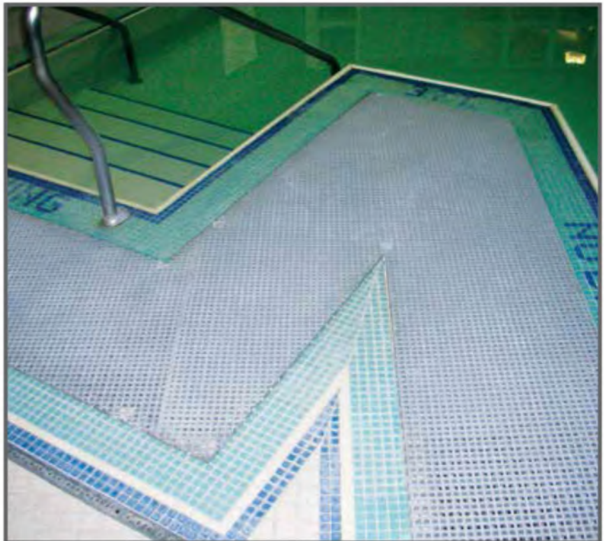
ZeAllgrate's Mini -Mesh molded grating, found in this public pool, required detailed fabrication due to the curves and angles of the pool's design.
