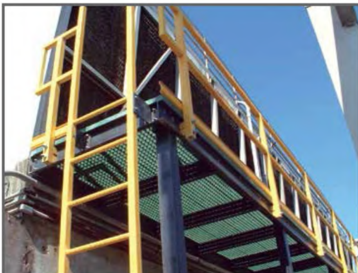
This all FRP structural system/platform uses ZeAll molded grating, railings and ladder, and FRP structural components. This engineered solution provides safe walkways for accessing cooling towers.
