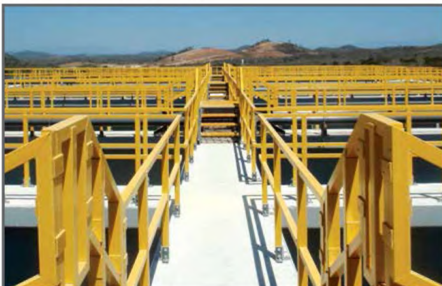
A partial view of miles of railing fabricated for a wastewater treatment facility in Mexico. This project also included several crossover platforms with stairways.
